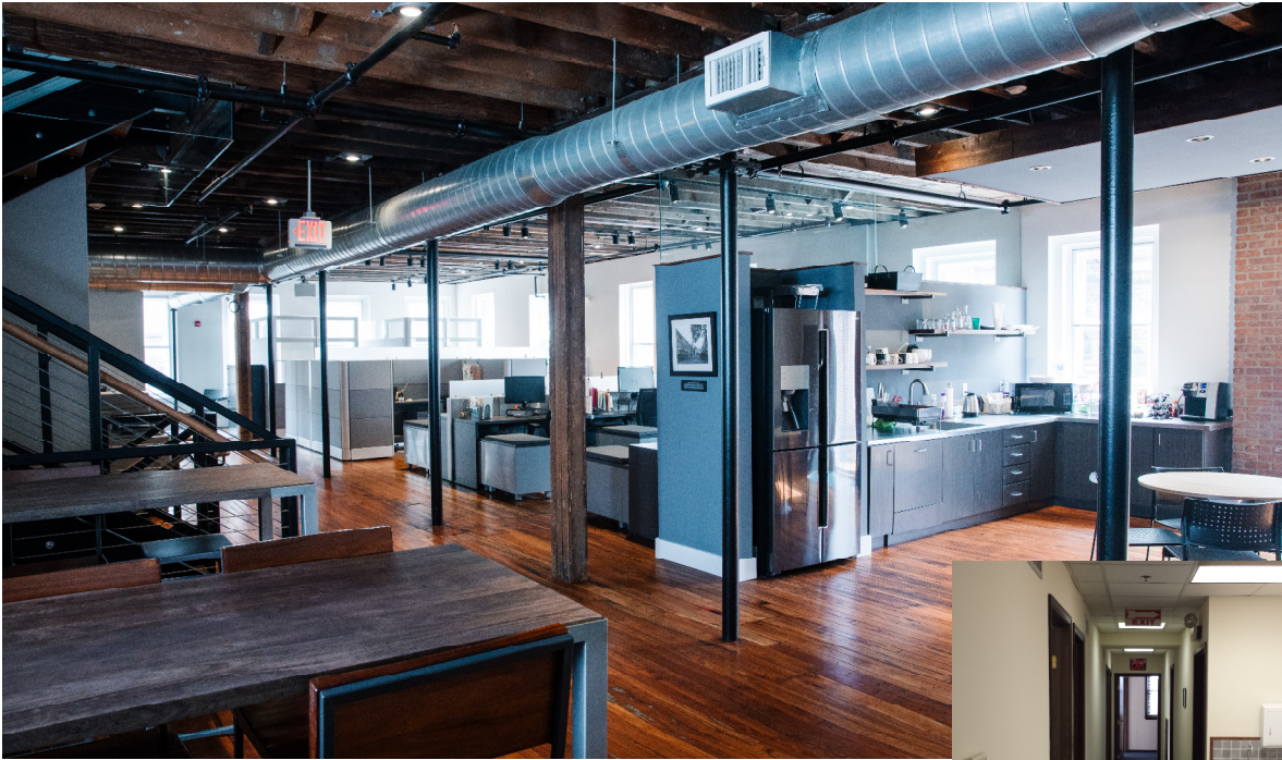
Above: Synchrony Group interior after renovation. Right: Before renovation Used with permission from Synchrony Group
