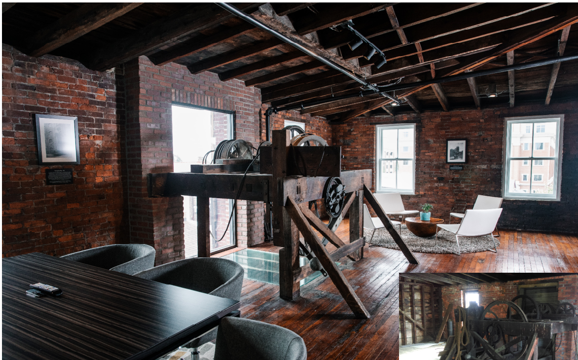
Above: Synchrony Group mezzanine after renovation. Right: Before renovation Used with permission from Synchrony Group Project Manager: Jeff Ivins, Dever Architects, 610-358-2300 jivins@deverarchitects.com
