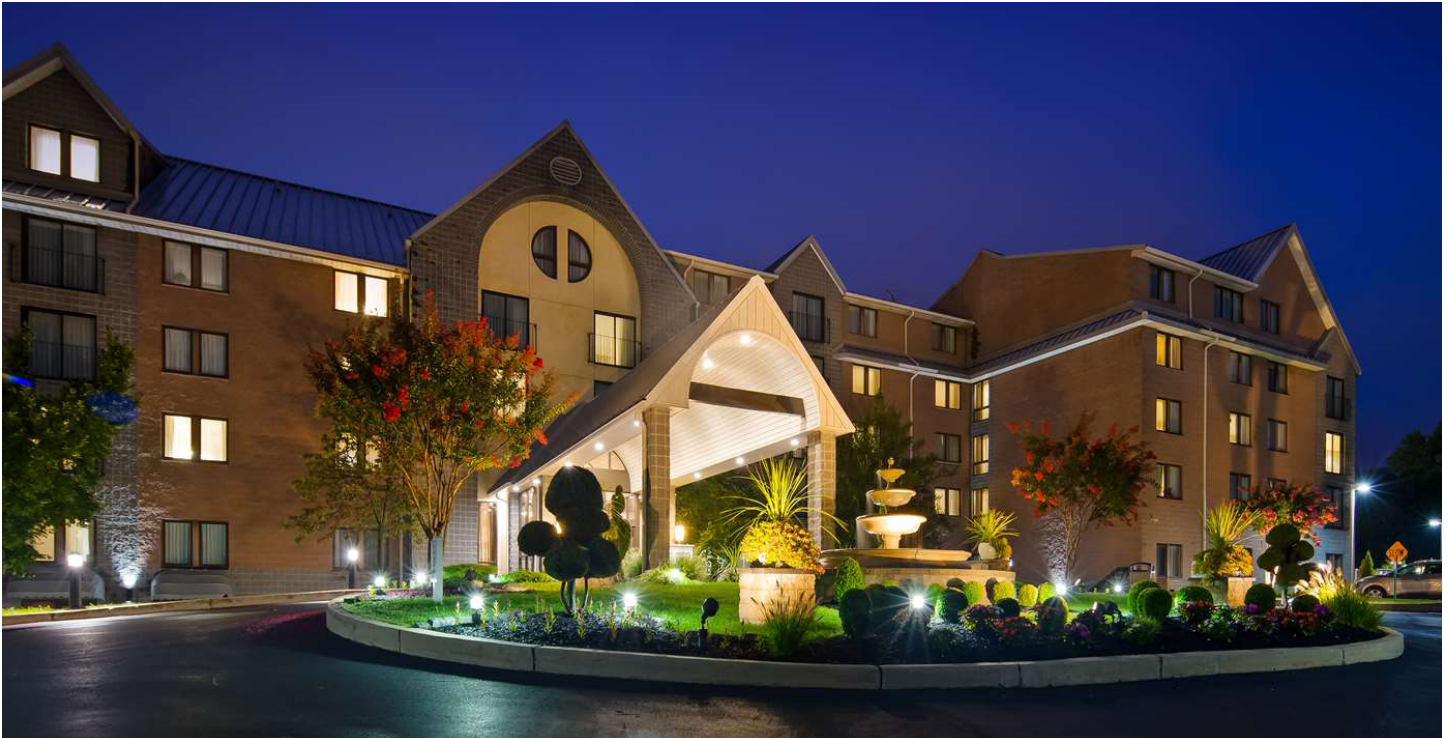
Above: "Concordville Hotel and Conference Center, built 1986" Photo from Best Western Hotels and Resorts
