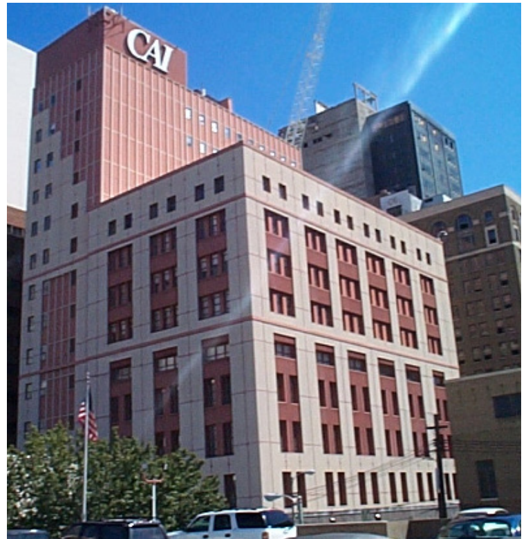
Previous Exterior from the 1980's Renovation
