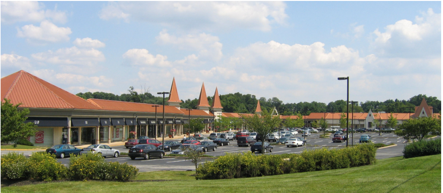
Above: "Glen Eagle Square, circa 2004" Photo from Dever Architects.
