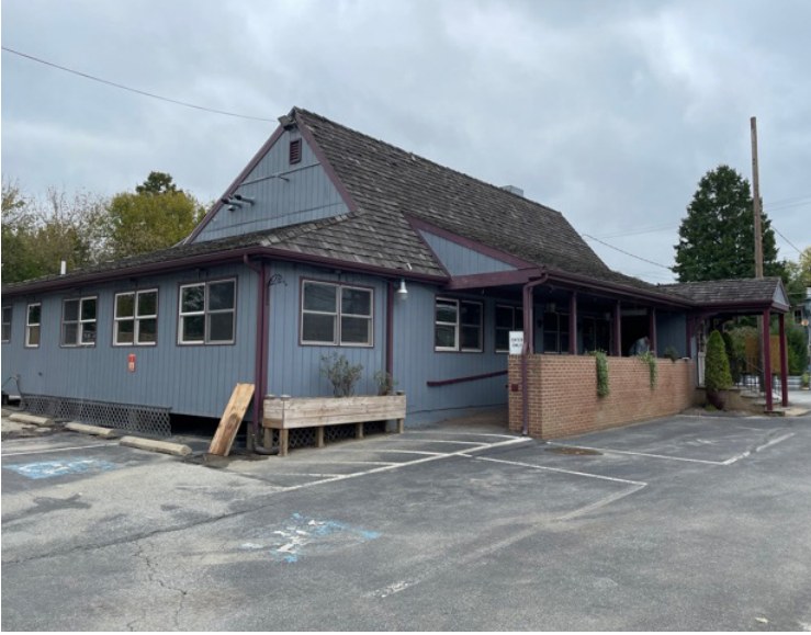
The building just after Hurricane Ida in 2021. Flood waters reached the ceiling! (Photo Courtesy: Dever Architects)
